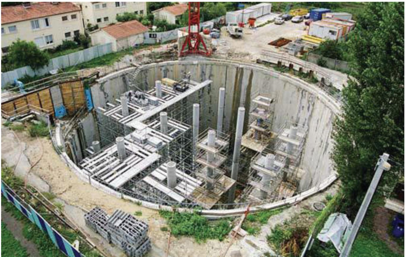
Diaphragm wall forms cylindrical shafts efficiently using the ordinary hydrofrises.
