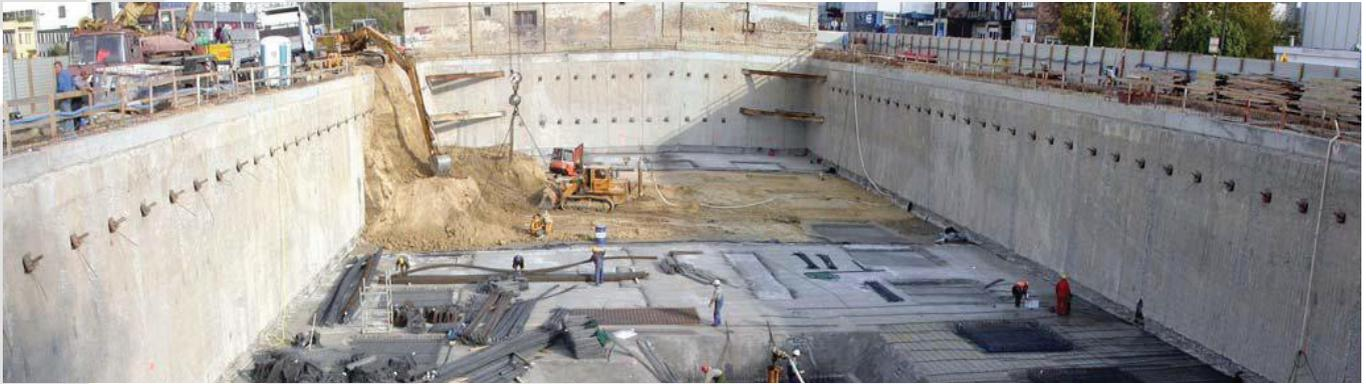
Diaphragm walls serve as shoring as well as permanent structural member. Raft foundation is proceeding in dry condition after completing the diaphragm (retaining) wall.
