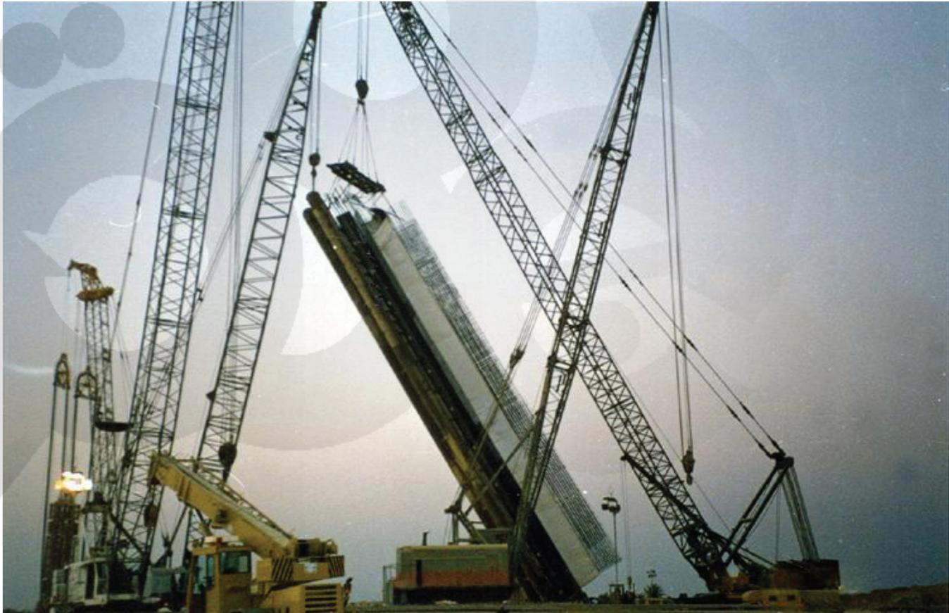
Three hydrofraises concurrently excavating diaphragm walls and barrettes while primary panel steel cage is lowered in a completed trench - North Ain Al Sukhna Port, Egypt
