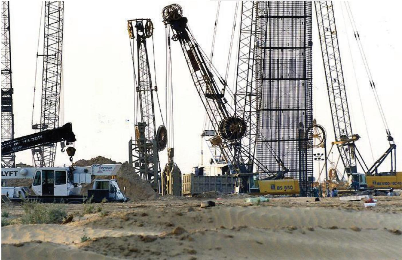
thickness and the interchangeable guide frames. The Hydrofraises (sometimes called hydromills) can meet walls design from 0.60m width and can exceed 2.0m width.
